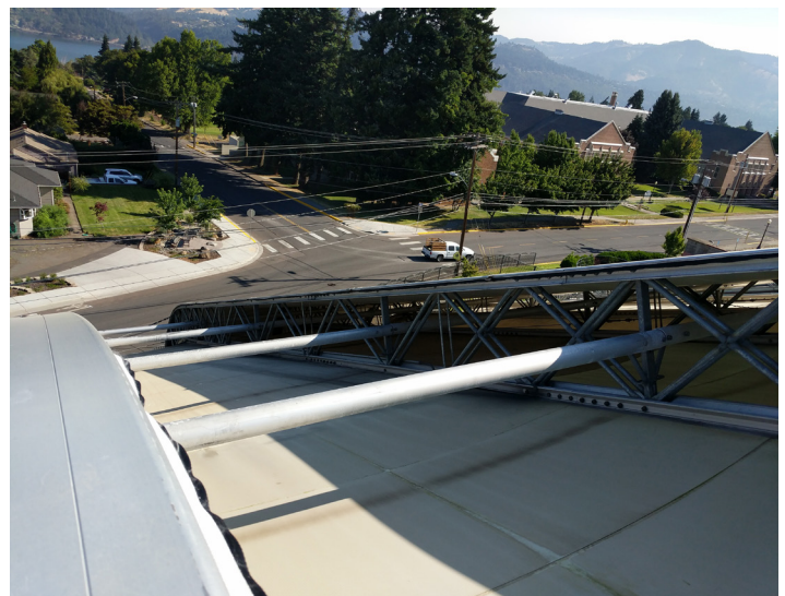
Emergency Panel Replacement: August 2017
